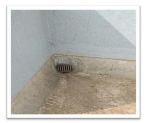
These photos can throw light on the proces of Rain Water Harvesting in college premises. Rain water from terrace passes through the pipes connected to terrace and stored in borewell. This water is utilized for washrooms and toilets. To aviod dust and blockages in pipes 2 nets are fixed and pebbles are put in chambers through which the water passes to borewell
